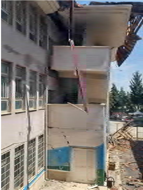
Fig. 10 Incipient (left) and total collapse (right) of the external structures bearing the emergency evacuation stairwells.
