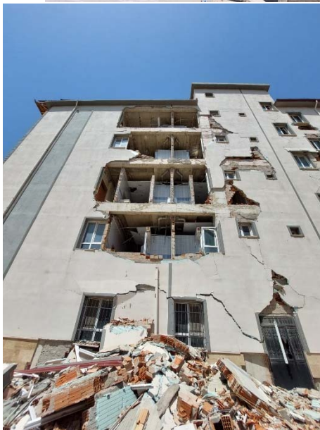
Fig. 5 Heavy damage of masonry infills, with out-of-plane collapse, corresponding to the front and back perimeter frames. Damage to the wooden roof cover with dislocation of roof tiles.
