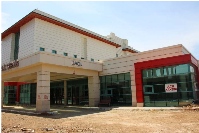
Fig. 13 – Existing hospital building built in 2012.
