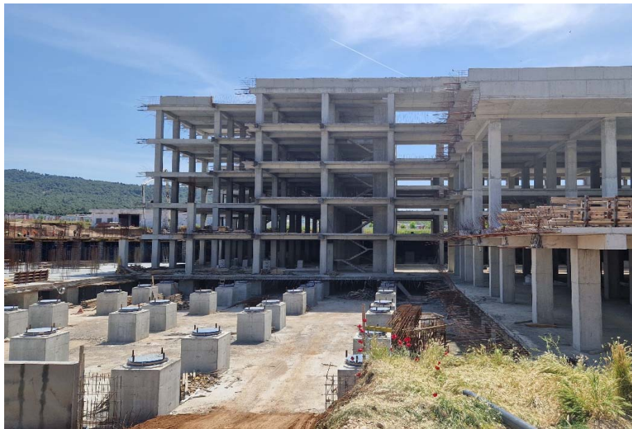
Fig. 12 – Side view of the structure under construction.
