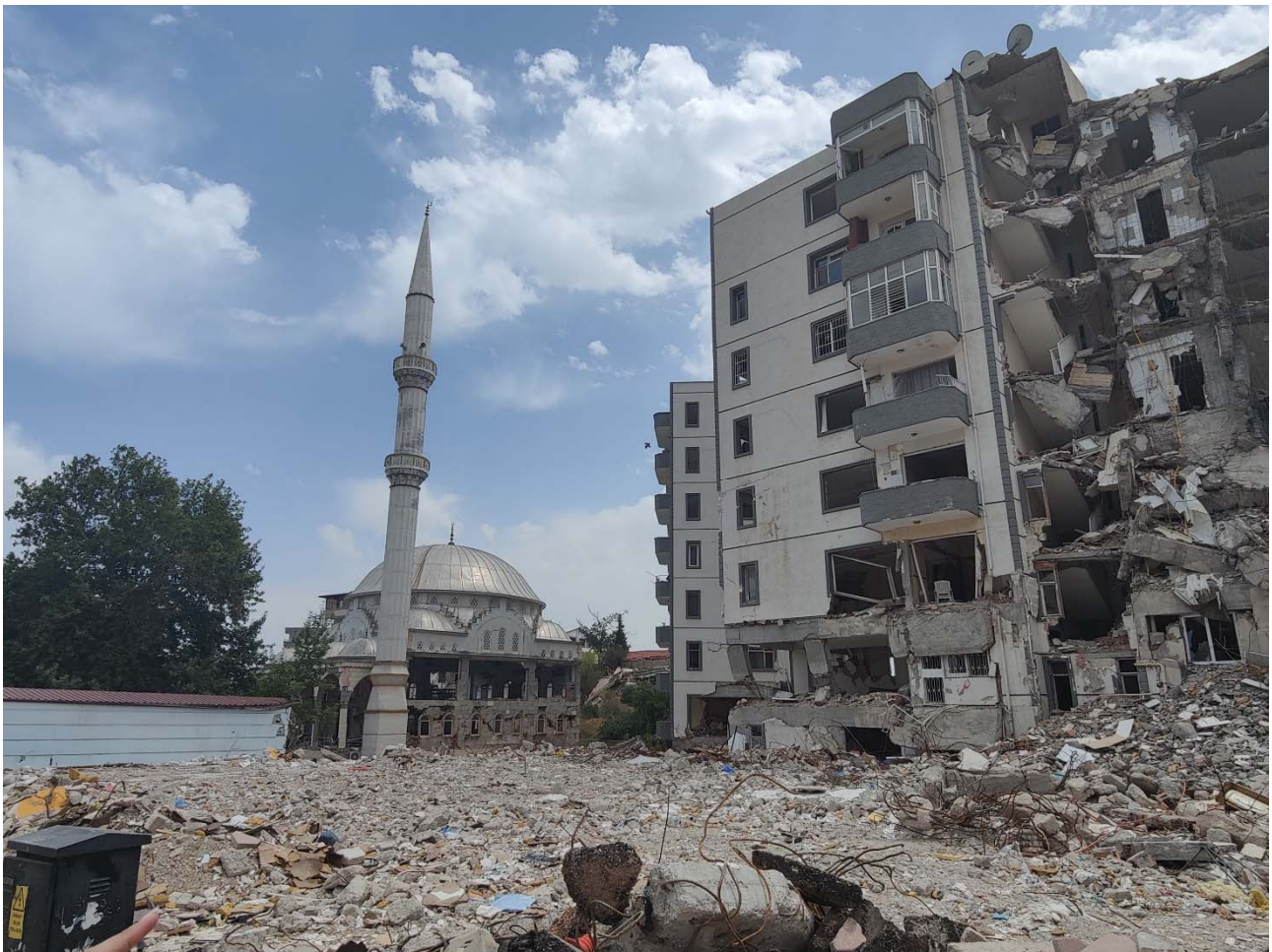
Fig. 10 – Residential complex in downtown Kirikhan.
