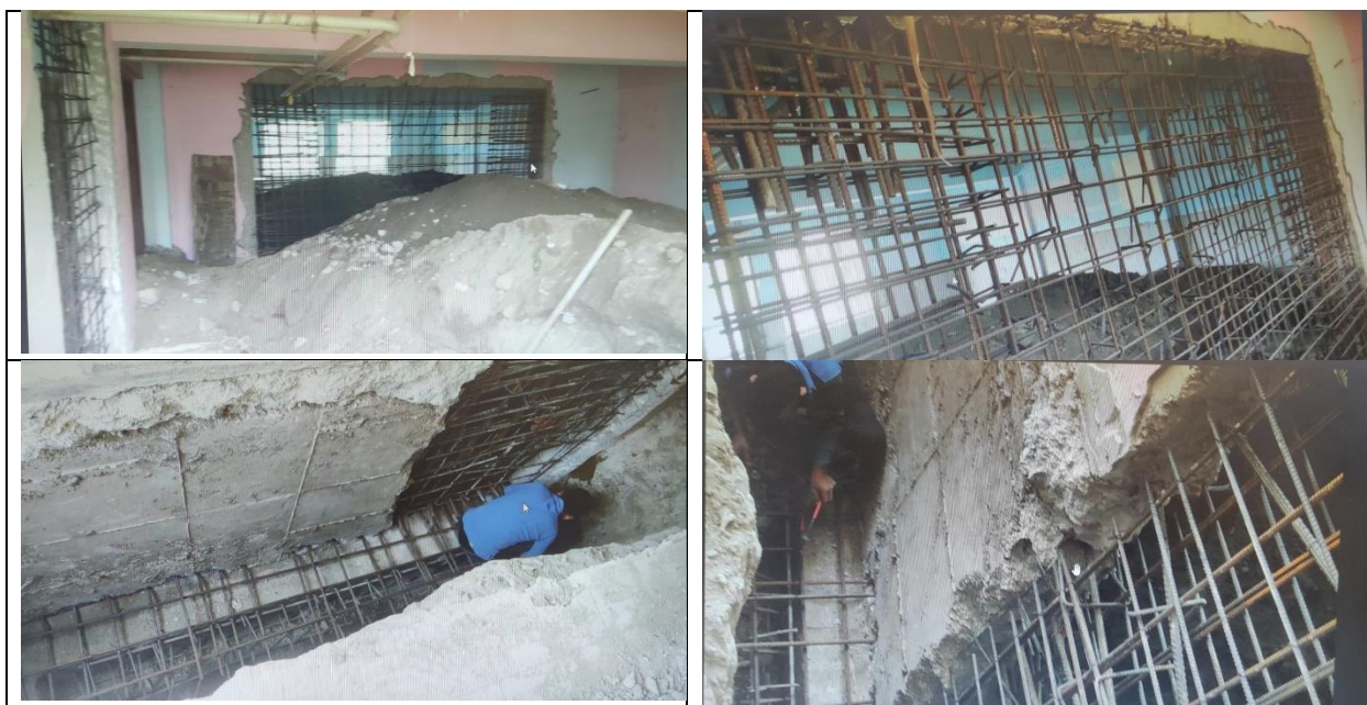
Fig. 5 – Retrofit works, still in progress just before the seismic event hit: excavation to foundation level for the needed upgrade in bearing capacity (a), removal of masonry partition in preparation for the addition of an RC wall and its integration into the surrounding frame (b, c).
