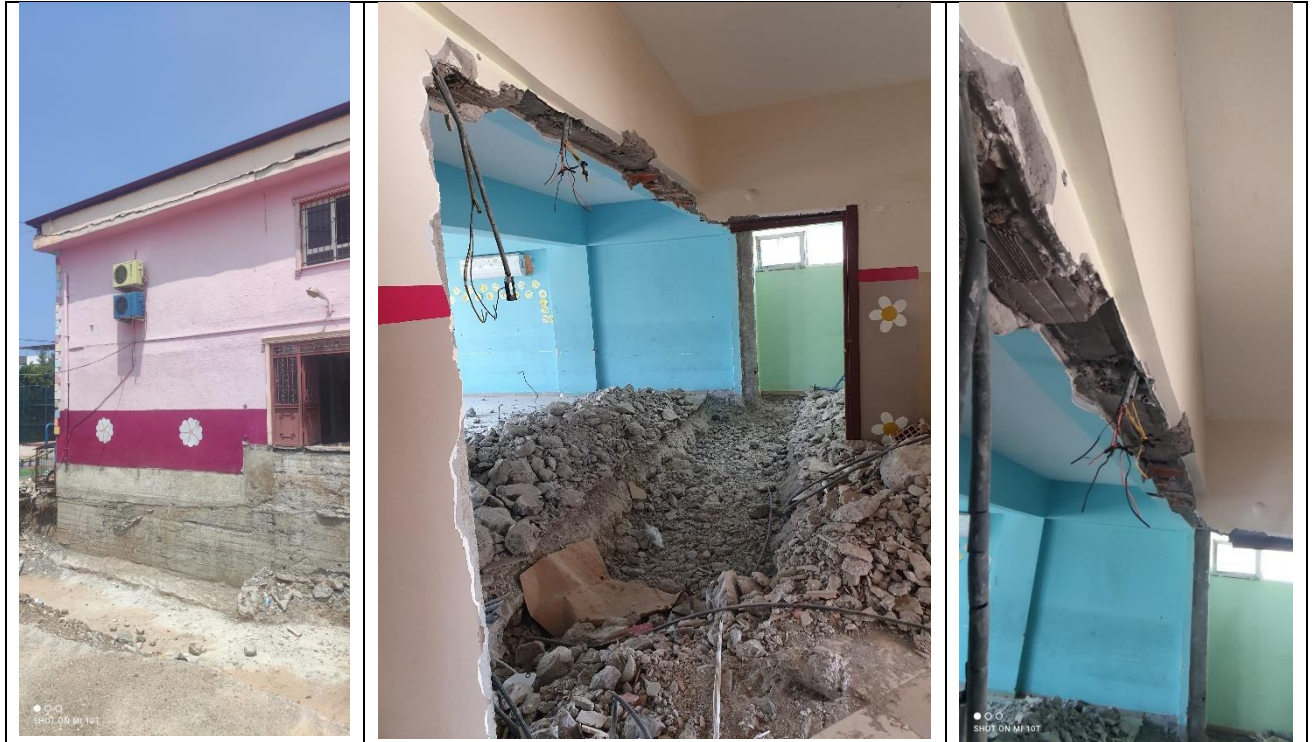
Fig. 5 – Retrofit works, still in progress just before the seismic event hit: excavation to foundation level for the needed upgrade in bearing capacity (a), removal of masonry partition in preparation for the addition of an RC wall and its integration into the surrounding frame (b, c).
